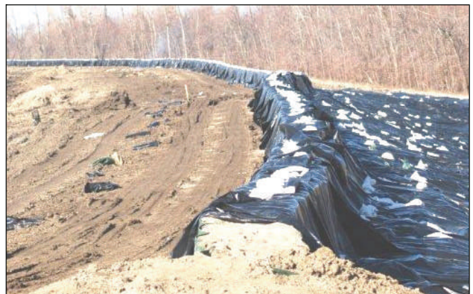
A completed section of levee at the upper crevasse Dec. 11. The plastic sheeting protects against erosion and provides a water-resistant barrier over the HESCOs.
