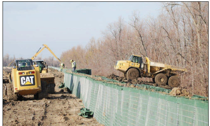
Crews fill HESCO barriers with sand at the upper crevasse Dec. 11. The temporary HESCO structure was completed Tuesday evening.
